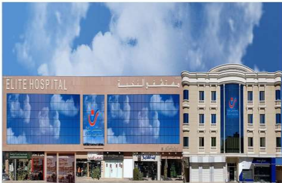
Elite Hospital Riyadh - KSA
